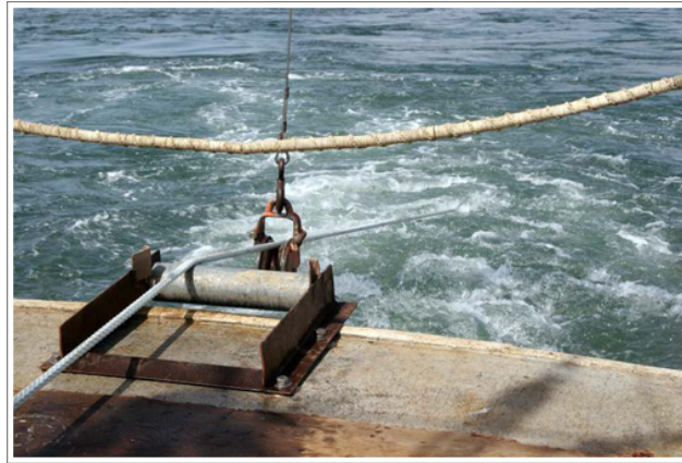
Figure 2. Anchor pull testing will be performed off a boat capable of deploying a 1 metric ton anchor, with instrumentation capable of determining pull loads for holding capacity estimates.
